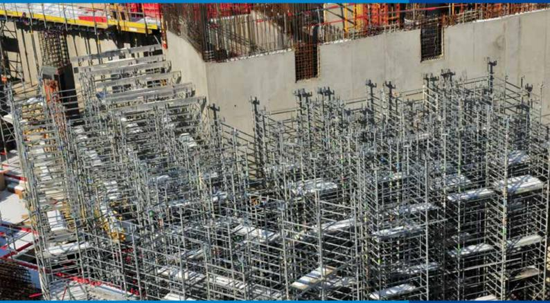
The A120 tower is a shoring tower that can be assembled and disassembled in complete safety. High-performance, it allows a load of 3 tonnes/foot.
