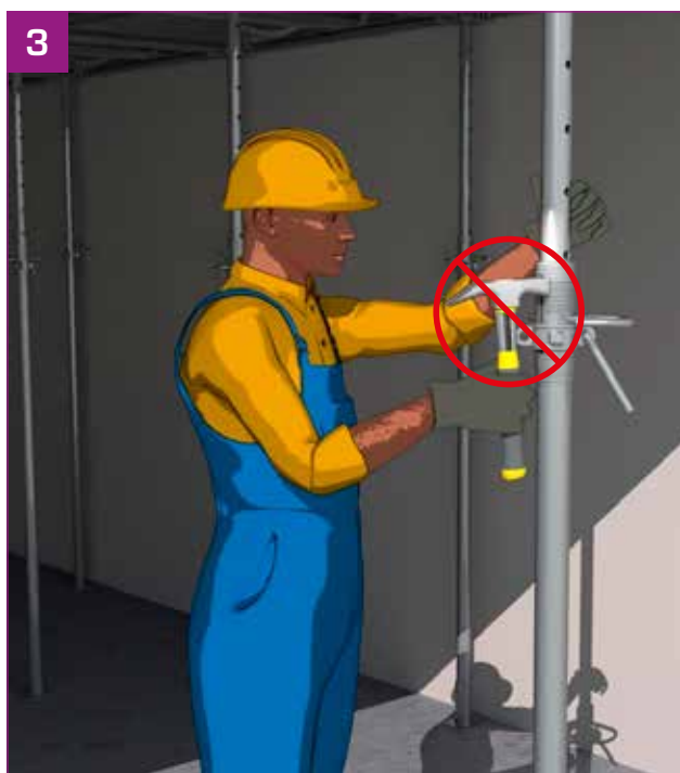
- Do not strike the threading with any tool liable to damage it.
